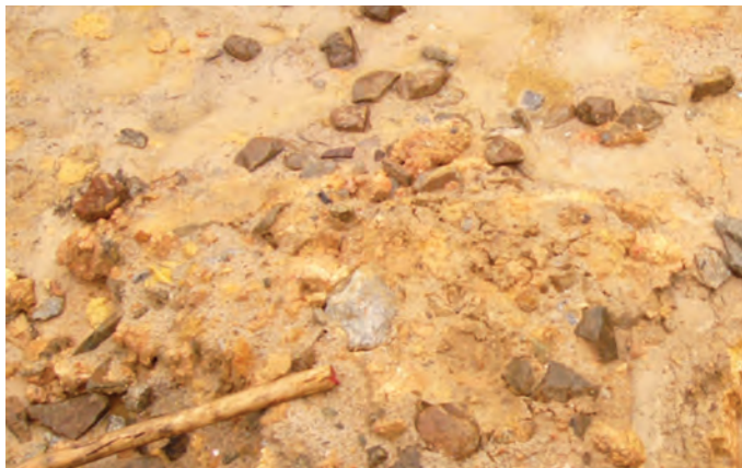
Fig 7. Rocks left during grading can interfere with subsequent drainage and aeration operations.
