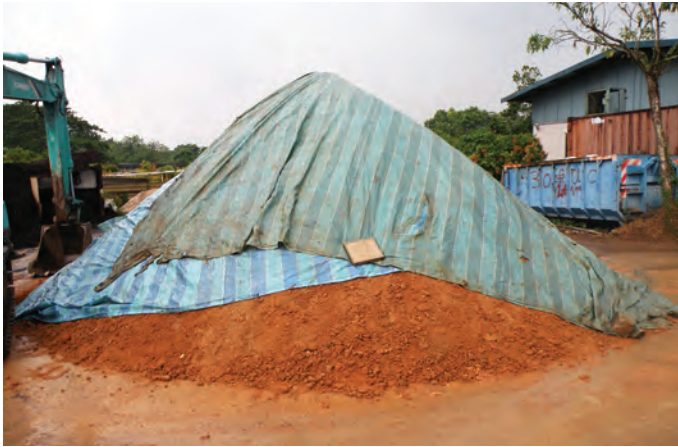
Fig 6. Stockpiling topsoil during the grading process.
